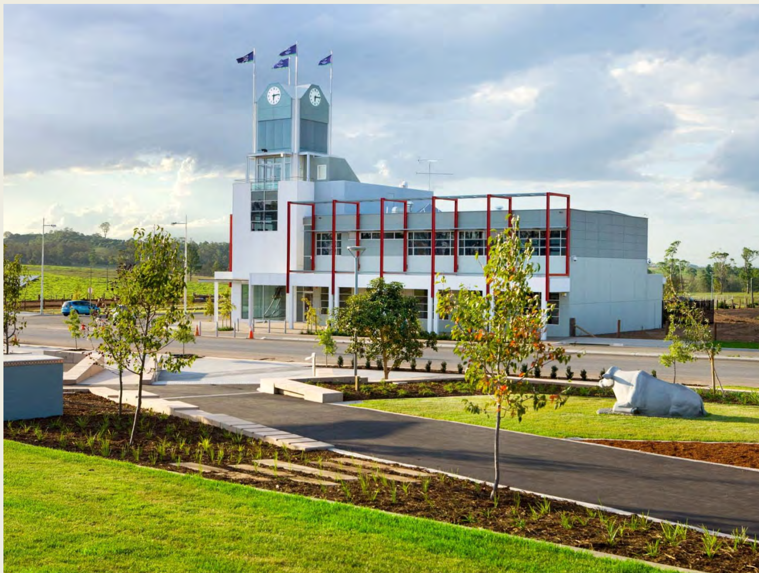
Oran Park Town sales and community centre
